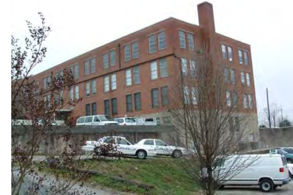
Existing Police Headquarters
