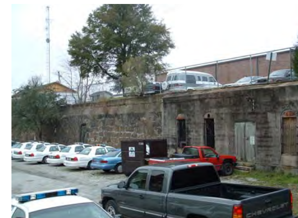
Historic Wall and Smith Shop behind Police Station
