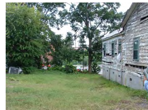
Existing housing and historic structure
